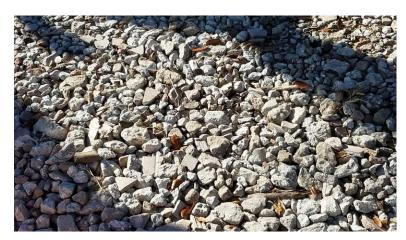
I inspected the recent repair on Wilderness Blvd. East to determine its readiness for paving. We will be replacing the top 6" with a finer grain of base material and then heavily compacting the repair area. The repair will be ready before the milling equipment reaches this area.
