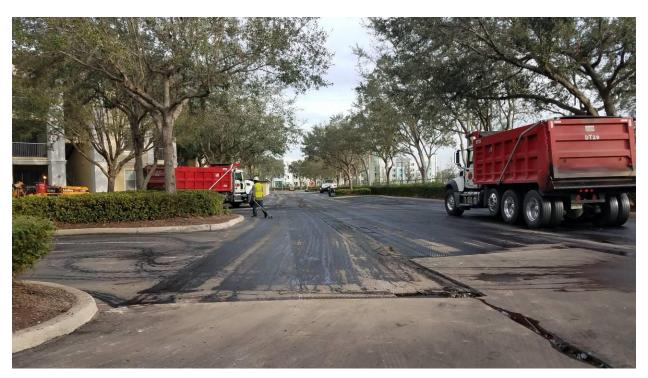
Another rumor that has surfaced is that the "tar" product will be applied after the milling and before the paving. This is true except that we are not applying the "tar"/tack until right before the paving machine. (see picture above from my last project) This product will be applied right before we install the asphalt and will take all of about 5 minutes to cure or "crack" and then within an hour or so, we will have the new asphalt in place. Within an hour of that we will
